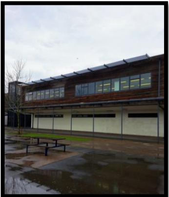
Whitecross Academy – Installation of New Canopy Structure
