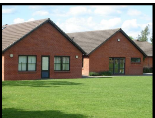
Lugwardine Primary School – Hall and Staff Room Extension
